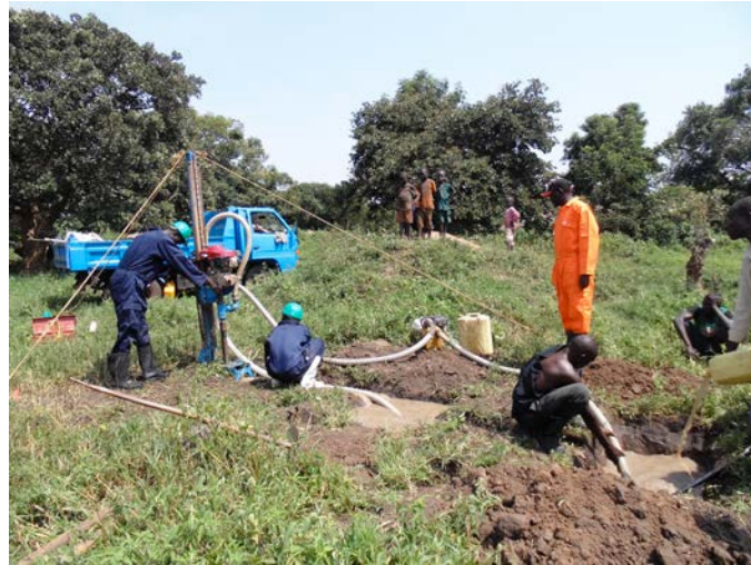
Drilling a well for a clean water supply for the village.
